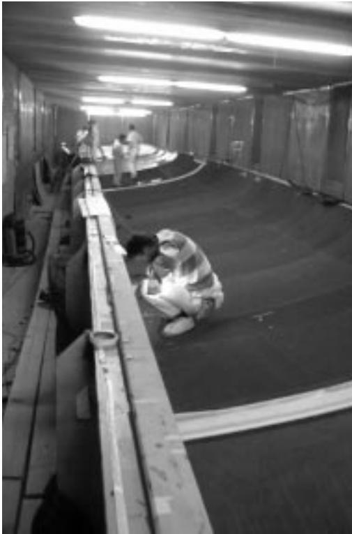
Pre-preg construction techniques inside one of the giant hulls
